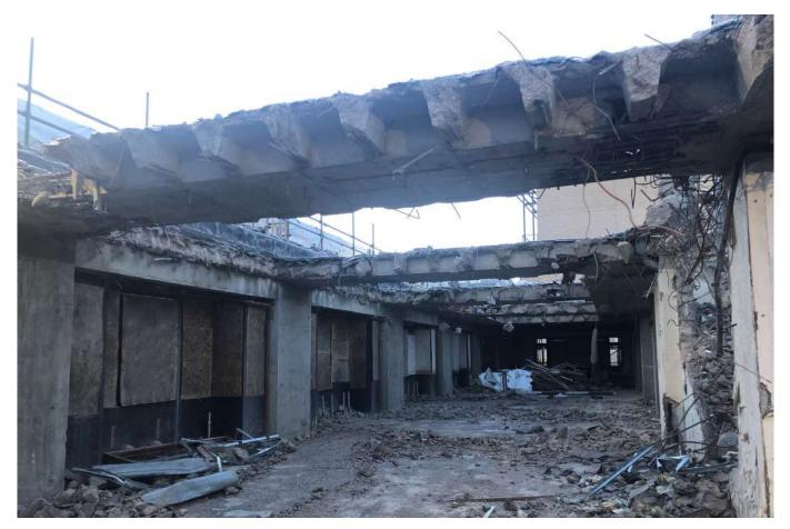
Framed systems can be constructed of steel or reinforced concrete. These may have infill panels of brickwork, blockwork, no-fines concrete, or precast concrete cladding.
