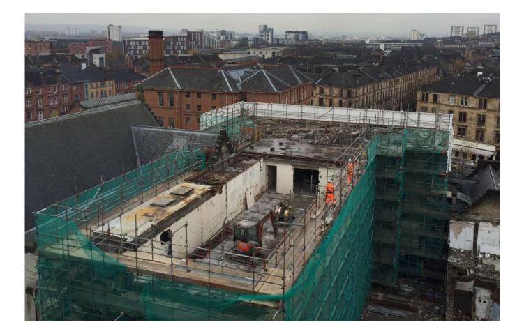
The erection and dismantling of all scaffolds (including ladder access) should be carried out by a competent scaffolding contractor and a formal handover certificate should be produced. The scaffold will be subject to continuous inspection throughout the works. Scaffold tagging systems should be used and seven-day mandatory inspections should be carried out throughout the works.
