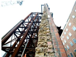
Loading of the temporary works should also be based around formal authorisation to load which may use a permit based arrangement. This can also be used to create hold points. An example of this would be the inspection of a propping scheme before the demolition moves onto the next bay.
